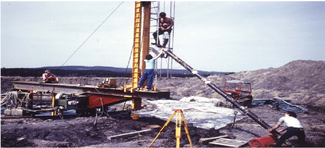
Figure 2.2.3- Picture from installation of test pile, Haga (from Karlsrud and Haugen, 1983)
