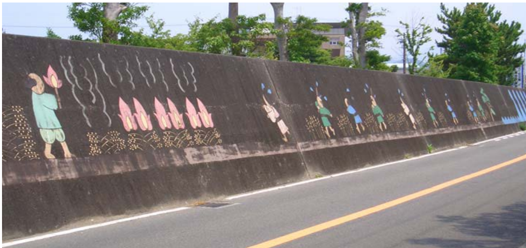
Dike in Hiro, Japan. Source: Ohta et al. 2005
