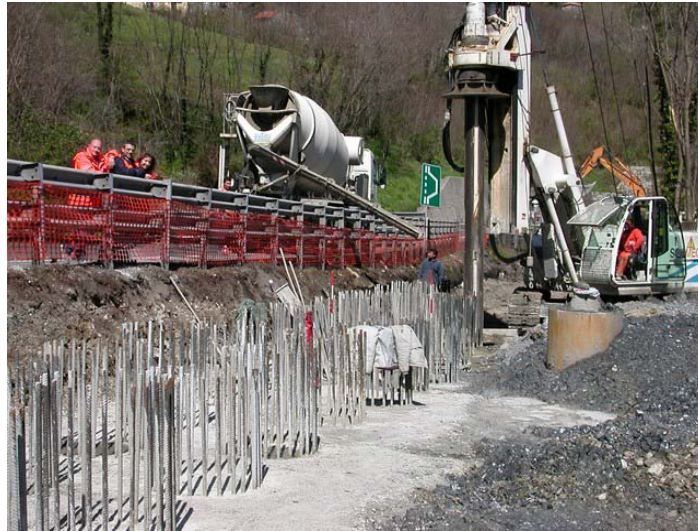
Figure 3.3.5 - Double row of large diameter piles
