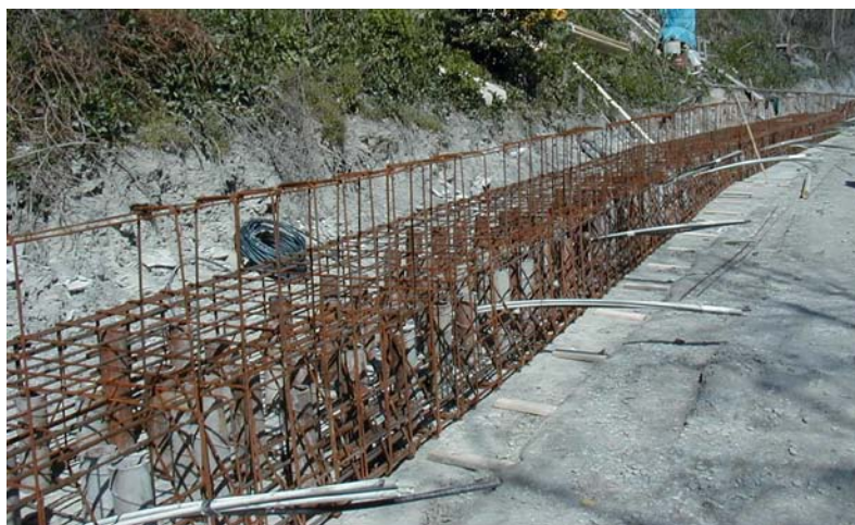
Figure 3.3.7 - Rows of micropiles reinforced by steel pipes
