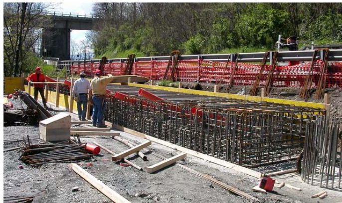
Figure 3.3.6 - Dapping beam connecting pile and anchor heads
