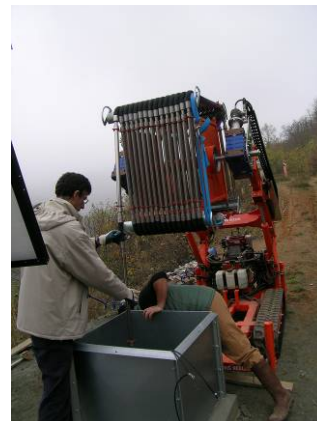
Fig. 3. Installation of D.M.S. column.
