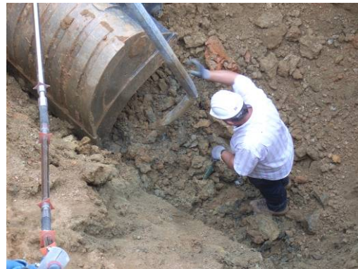
Fig. 9. Removal of D.M.S. column.
