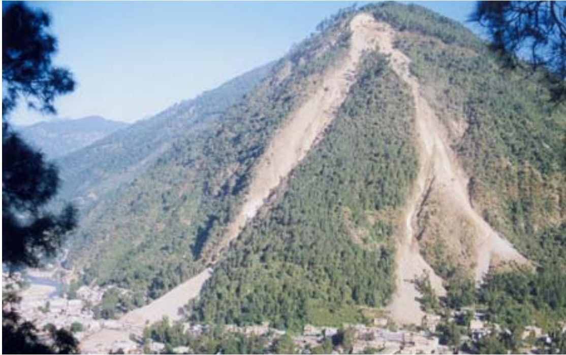
Figure 3. A panoramic view of Varunavat landslide, Uttarkashi
