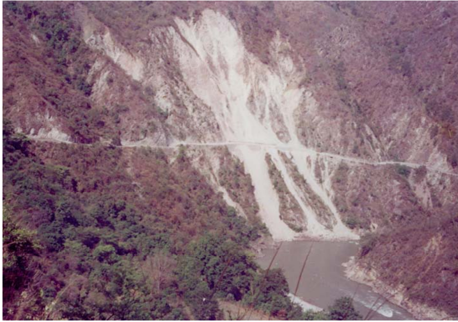
Figure 14. Frontal face of the Kaliasur landslide
