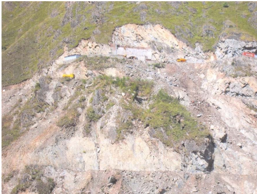
Figure 30. The NTPC landslide
