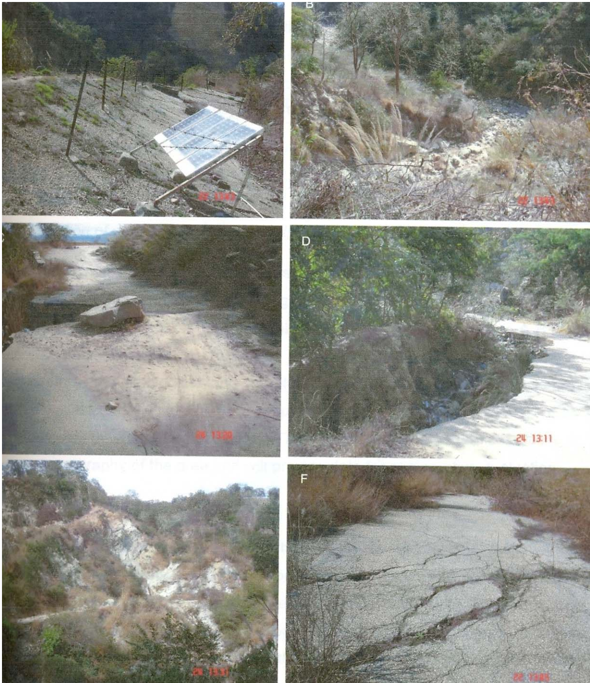
Figure 31. Mansadevi landslide and its impact
