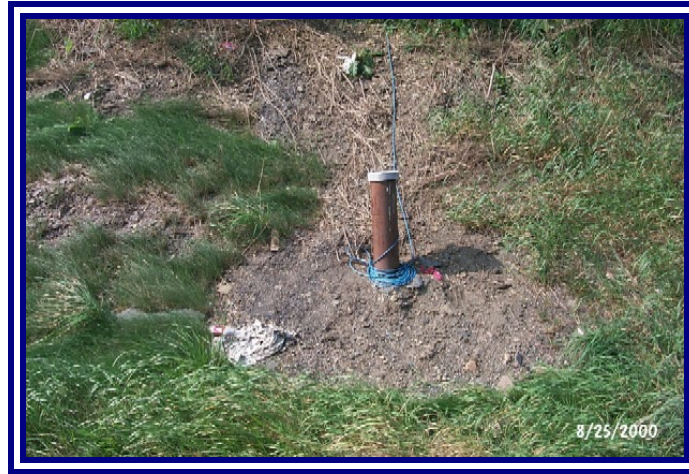
Figure 10. A Tiltmeter installed underground
