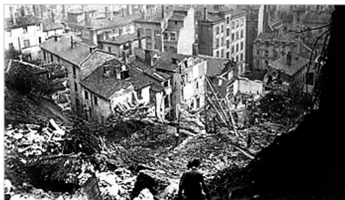
Figure 4.4.1 View of the Fourvière slide (Ref: http://www.musee-pompier.aso.fr/ )
