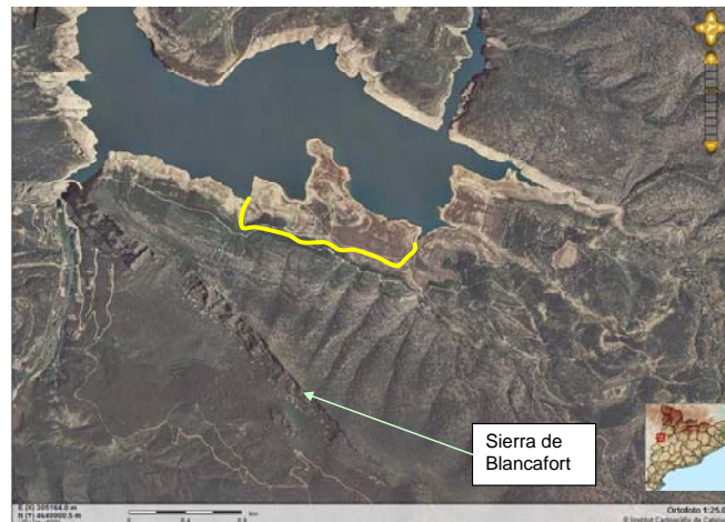
Figure 4.3.1 Aerial view of Canelles reservoir. Landslide contour indicated by the yellow line (approximate length of yellow line: 1.8 km).
