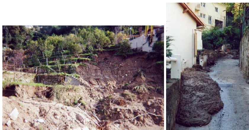
Figure 4.8.2 View of shallow landslides and mudflows
