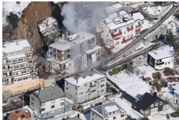
Figure 4.6.1 View of the Aalesund slide (ref: Skredulykka I Aalesund, 2008)
