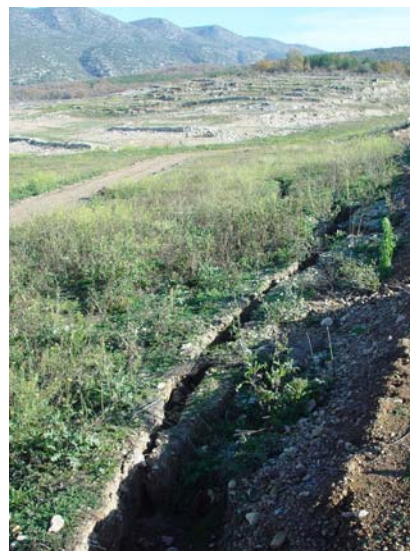
Figure 4.3.2 Detail of a tension crack at the foot of an ancient scarp. The motion of the slide (on the left) looks essentially translational.
