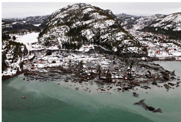
Figure 4.7.1 View of the Namsos slide (Photo by Leif Arne Holme)
