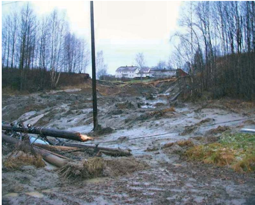
Figure 19. Landslide at Dorr, Minnesund, South-Eastern Norway triggered on 22 November 2000 (Jaedicke and Kleven 2008).
