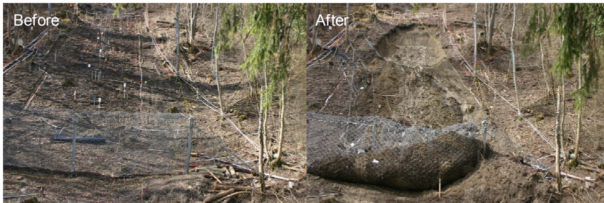
Figure 9- Rüdlingen slope: before and after failure on 17 th March.
