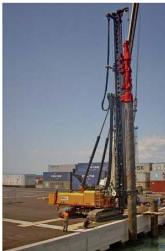
DELMAG diesel pile hammer D46-32 on piling rig BANUT 655 in Slovenia
