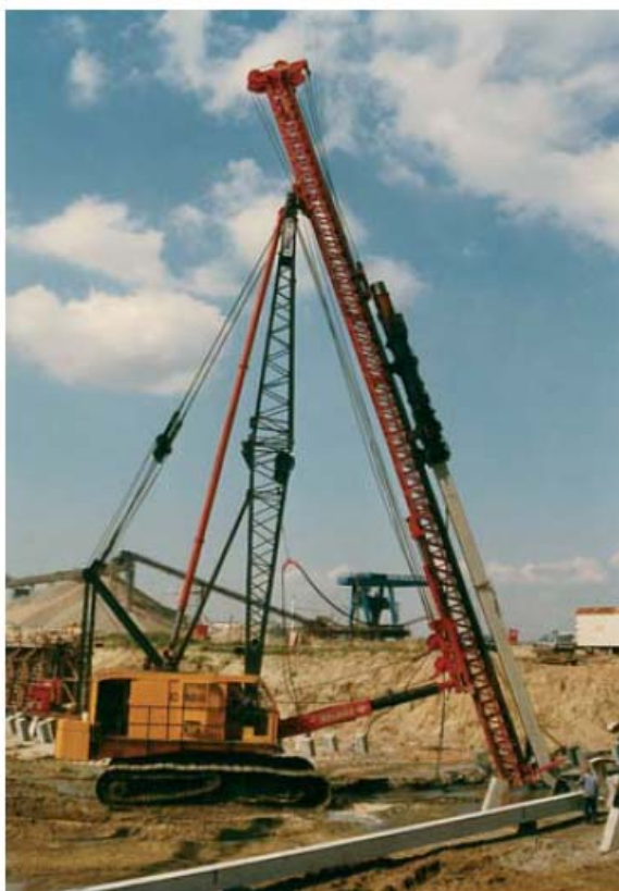
DELMAG diesel pile hammer D62-22 on hanging lead MH 8007 in Belgium
